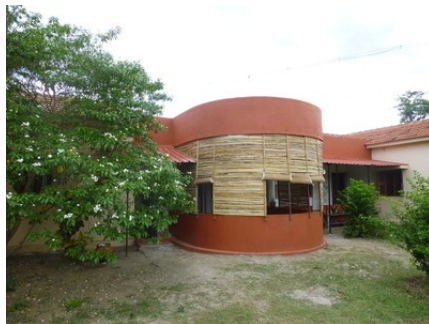
The temporary nursery school building
